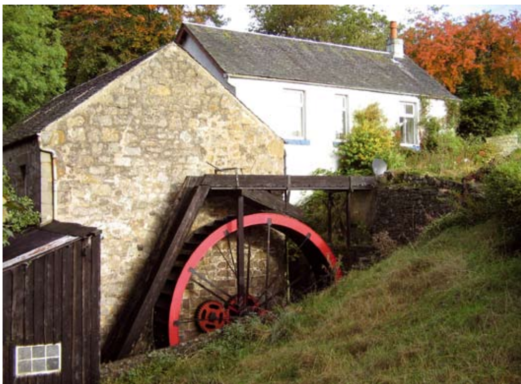
Figure 2. Baldernock Mill from the south. The white rough-cast building on the right is a mid-19th century dwelling built over the remains of the mill's drying kiln. The stone building in the centre is the corn mill building, and the dark timber building lower left is the lean-to saw mill, which is still operational. The mill wheel is pitchback with the lade delivering water from the right (from the upstream dam) and the water flowing back to the right from the gently sloping wooden box channel (the launder), down the right-sloping steep chute to drive the wheel. The long steep left-sloping structure to the left of the wheel returns unused water from the lade to the burn, lower left. The masonry wall at the mill wheel (the so-called water wall) bears circular scratch marks from an earlier, smaller diameter wheel
